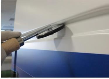
Important: In order to avoid lifting at the overlaps of the panels, post-heating of the overlaps with the hot-air gun up to +120°C is necessary to avoid lifting failures.
